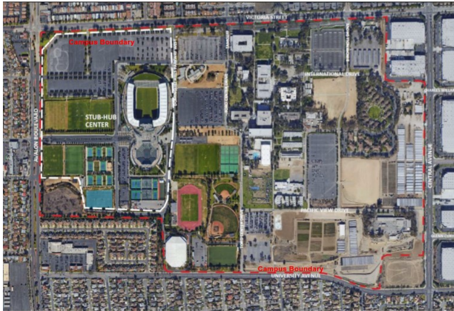
Figure 3.7-1 Aerial Photograph of CSU Dominguez Hills Campus, 2016
