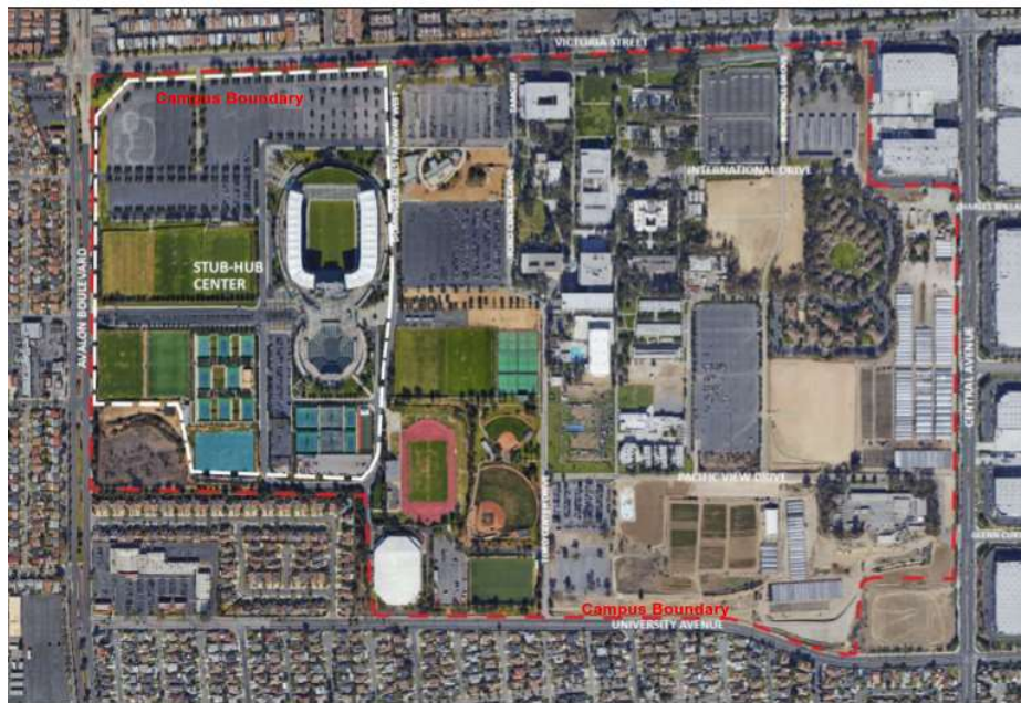
Figure 3.9-1 Aerial Photograph of CSU Dominguez Hills Campus 2016
