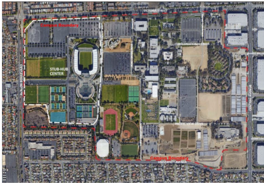
Figure 3.6-1 Aerial Photograph of CSU Dominguez Hills Campus, 2016
