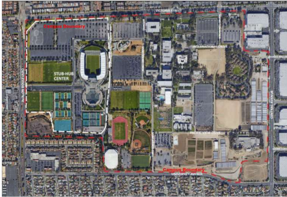
Figure 3.10-1 Aerial Photograph of CSU Dominguez Hills Campus, 2016
