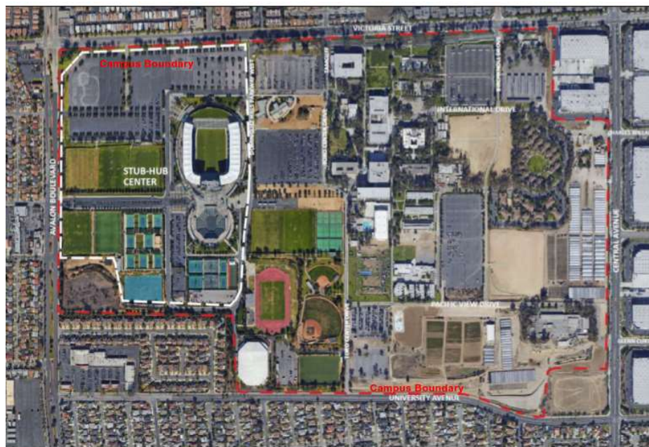
Figure 3.4-1 Aerial Photograph of CSU Dominguez Hills Campus, 2016
