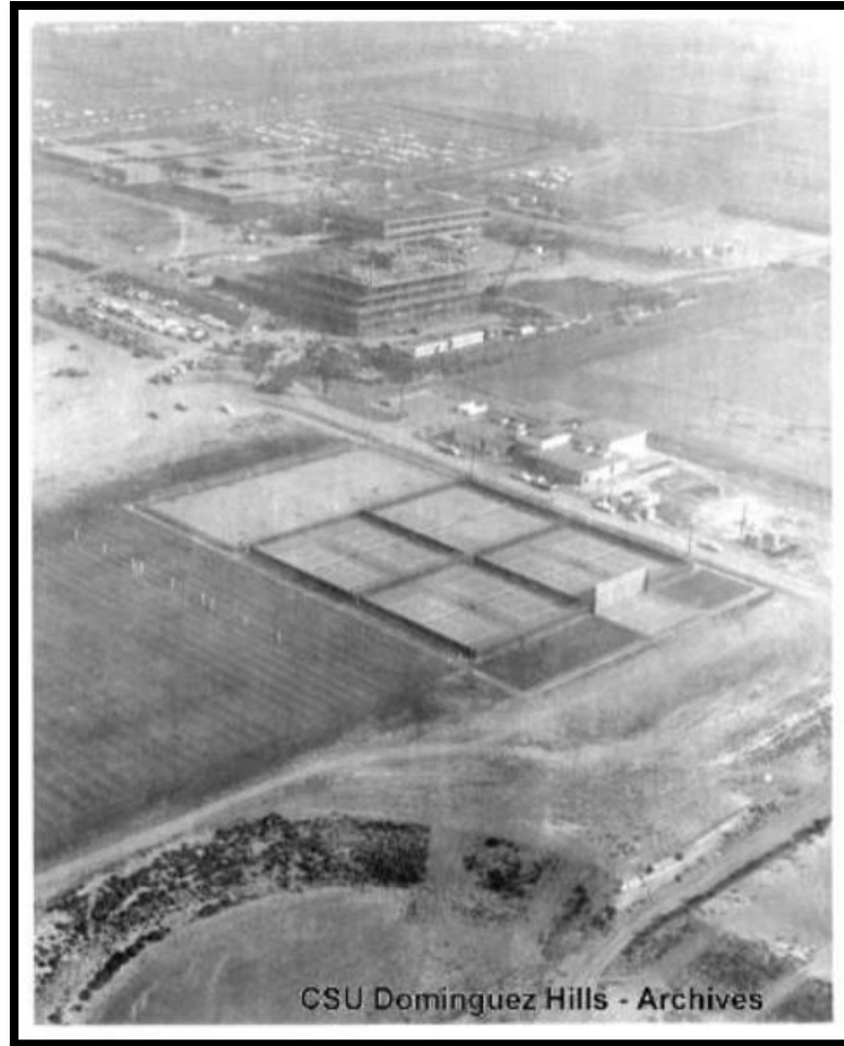
Figure 1. Campus Construction, c. 1970. The Small College Complex is located at the top of the photo and the Leo F. Cain Library/Educational Resource Center is under construction.
