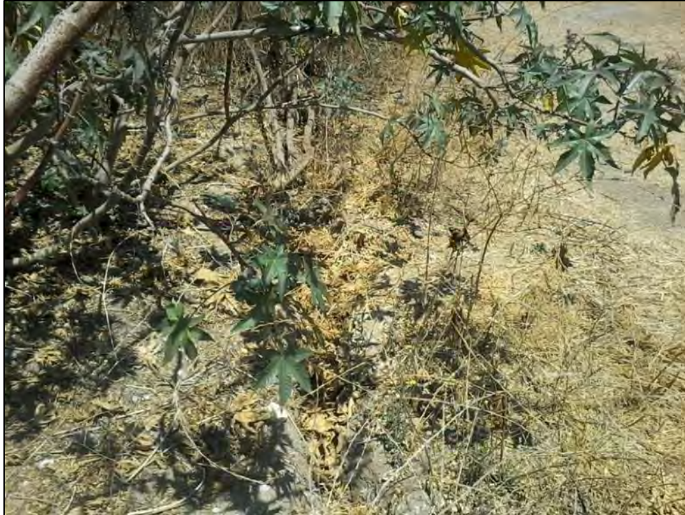
PHOTO 31. DRAINAGE SOUTH OF THE PHYSICAL PLANT, FACING WEST.
