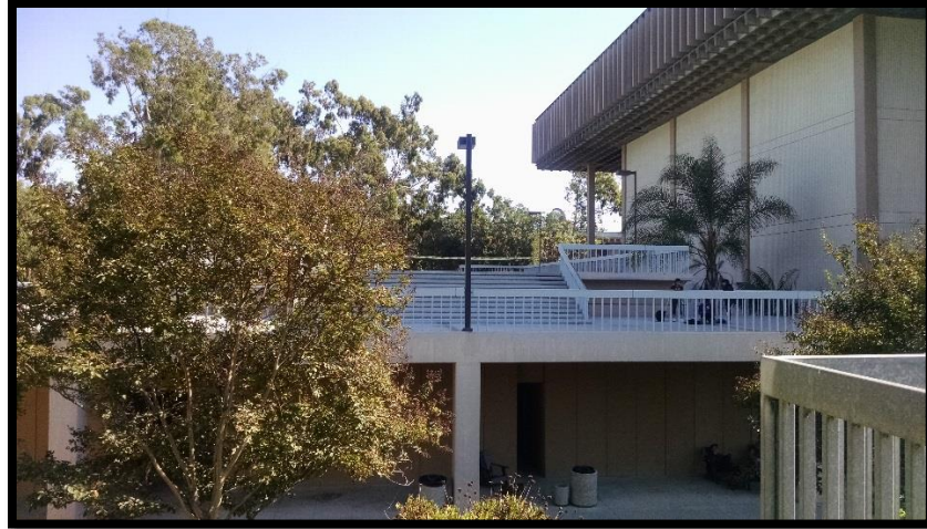
Figure 9. View east toward library facade and sunken courtyard.
