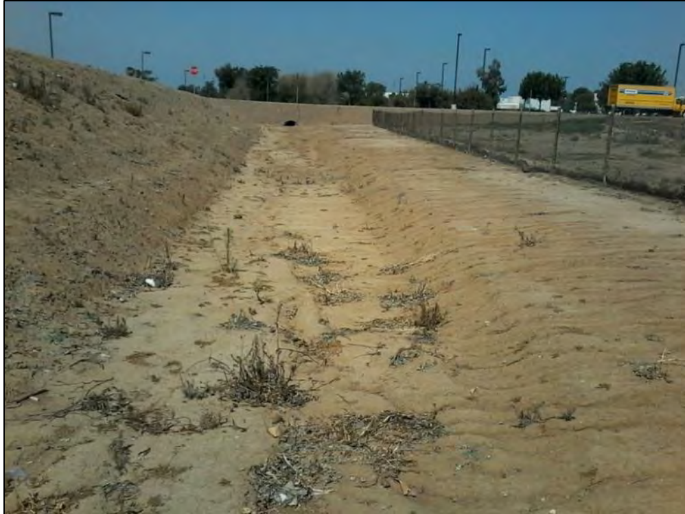
PHOTO 19. DRAINAGE LOCATED ALONG PACIFIC VIEW DRIVE, FACING WEST.
