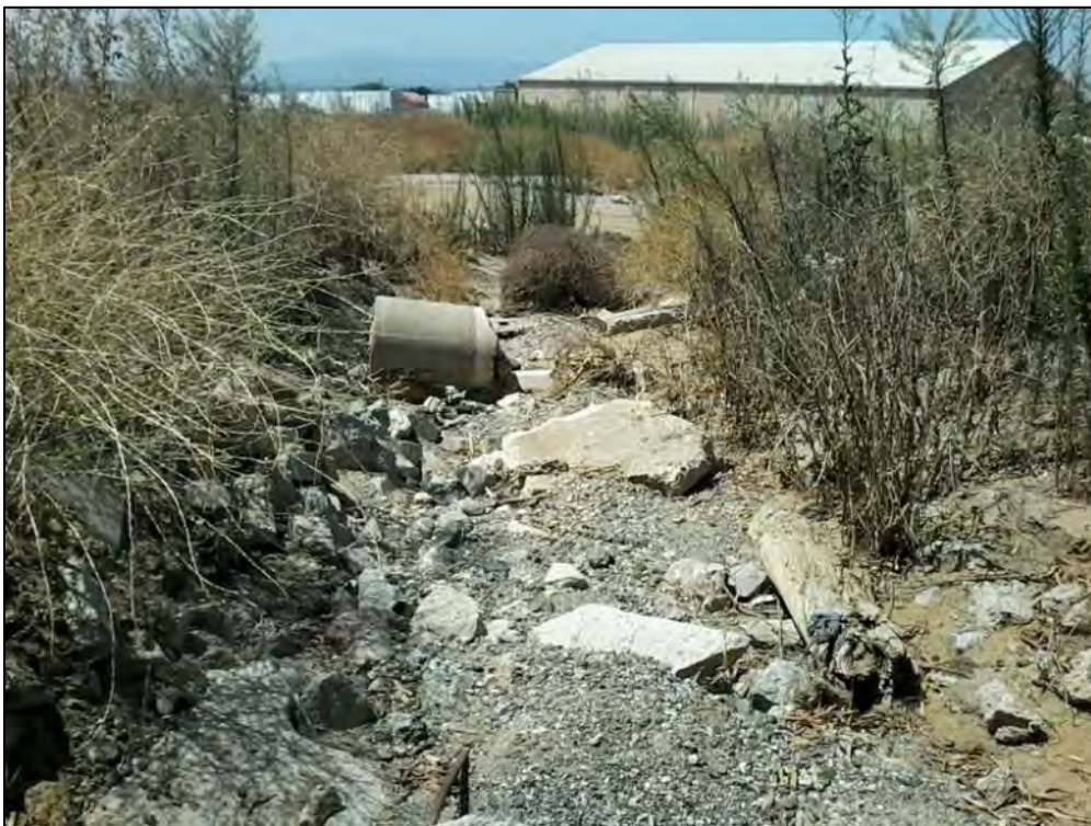
PHOTO 26. DRAINAGE WEST OF THE PHYSICAL PLANT, FACING SOUTHWEST.
