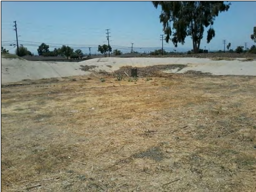
PHOTO 24. DRAINAGE WITHIN DETENTION BASIN SOUTHWEST SIDE OF MAINTENANCE FACILITY, FACING SOUTH.
