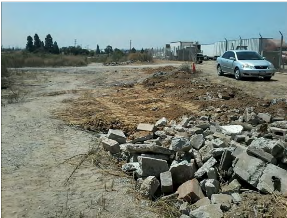
PHOTO 28. FILLED DRAINAGE EAST OF THE MAINTENANCE FACILITY, FACING SOUTH.
