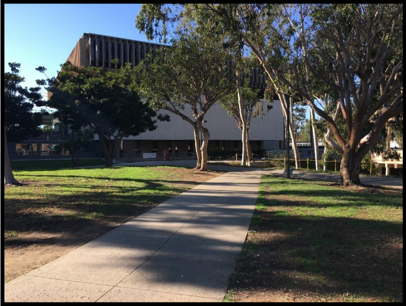
Figure 8. View west toward library's east elevation.
