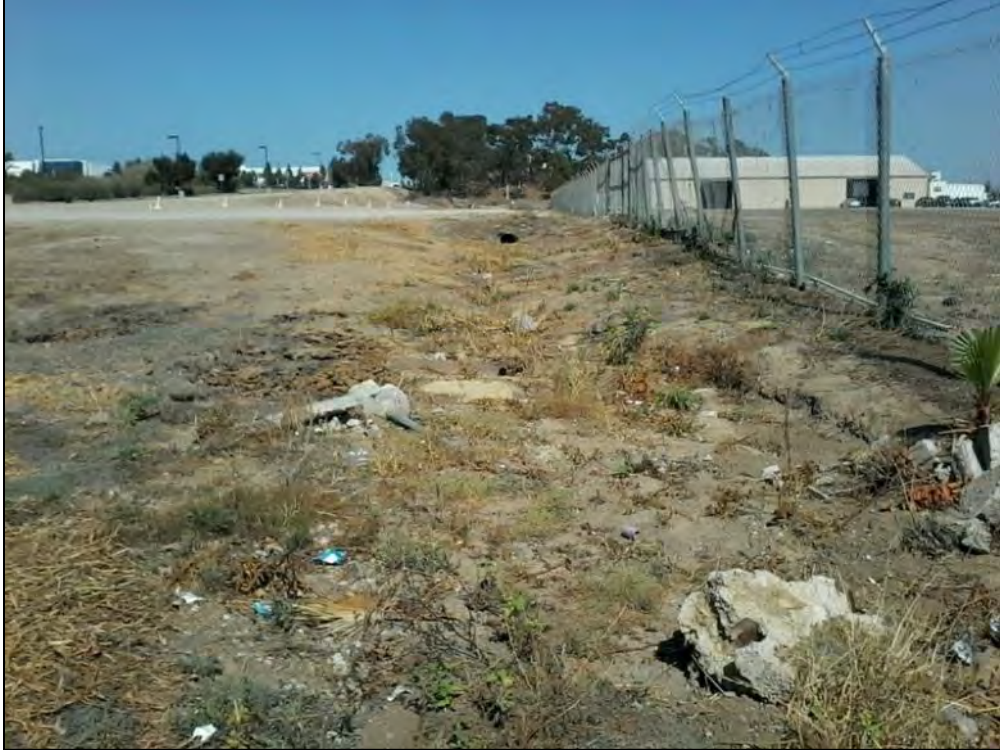
PHOTO 21. DRAINAGE LOCATED ON NORTH SIDE OF MAINTENANCE FACILITY, FACING EAST.
