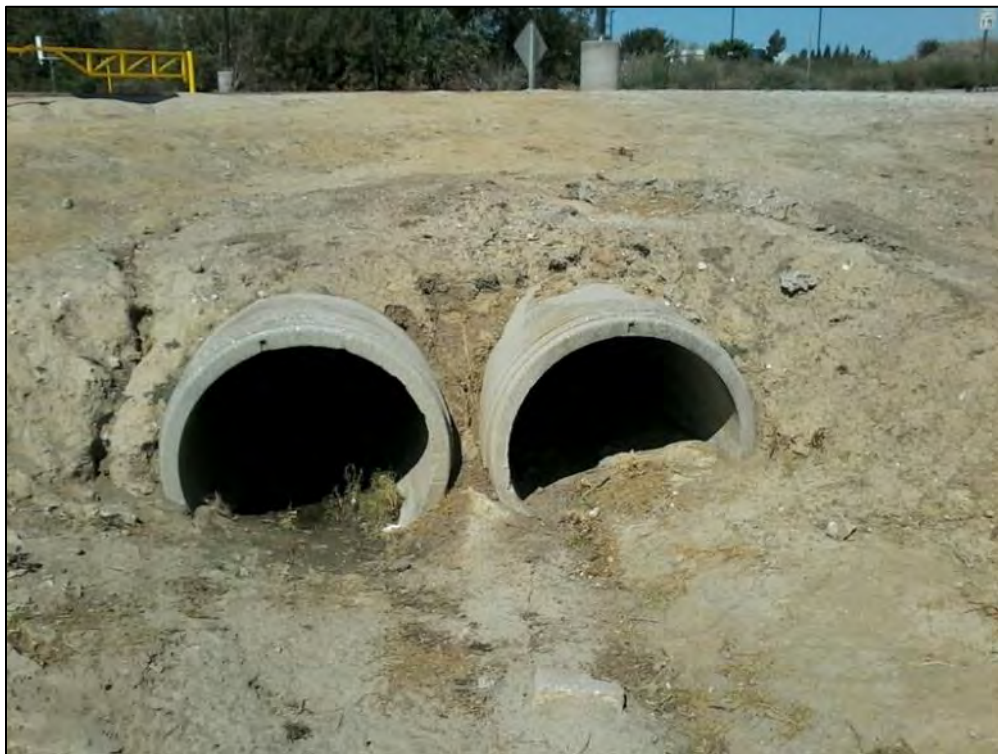
PHOTO 20. CULVERTS ON DRAINAGE LOCATED SOUTH OF PACIFIC VIEW DRIVE, FACING NORTH.
