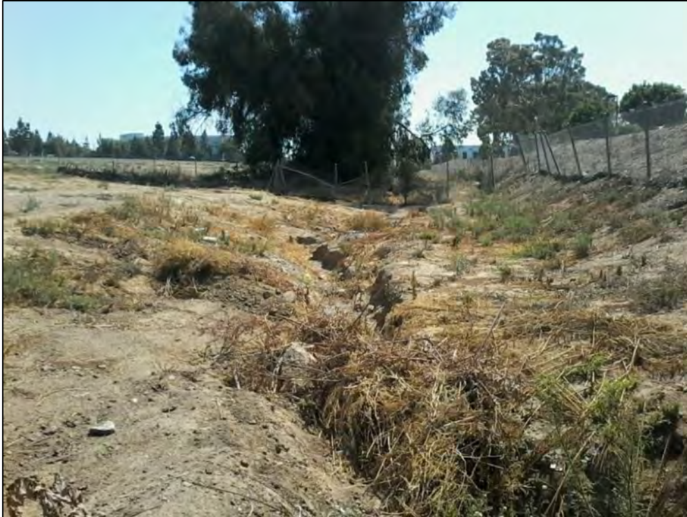
PHOTO 25. DRAINAGE NORTH OF THE PHYSICAL PLANT ALONG PACIFIC VIEW DRIVE, FACING EAST.
