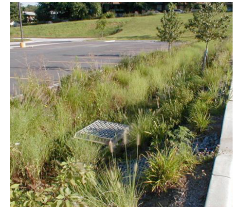
Exhibit 6-15: Bioswale with Filtration Vault
