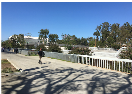
Exhibit 7-12: East Walkway railing
