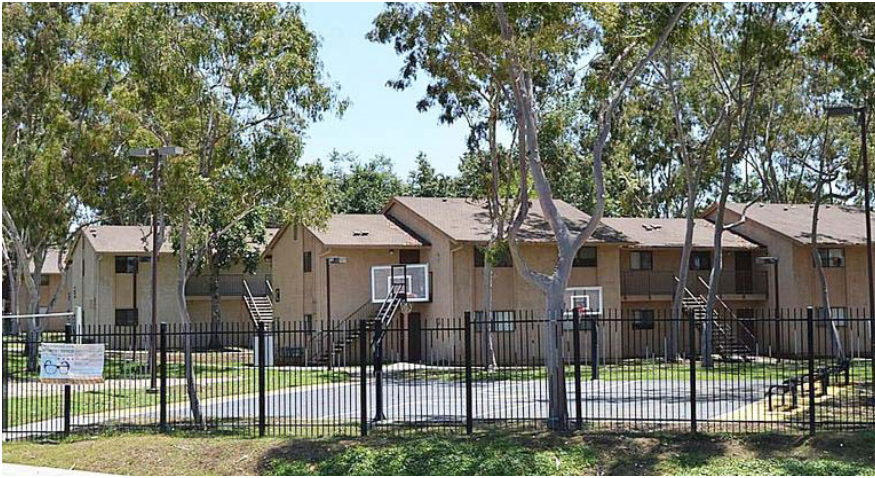
Exhibit 1-5: One Master Plan Goal: Increase Campus Housing. (Pictured: CSUDH Pueblo Dominguez Student Housing)
