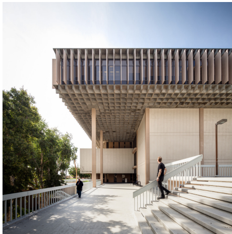
Exhibit 7-3: Original structural system (Leo Cain Library)
