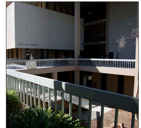
Exhibit 5-6: Railings adjacent to Leo. F Cain Library, with view into lower level courtyard
