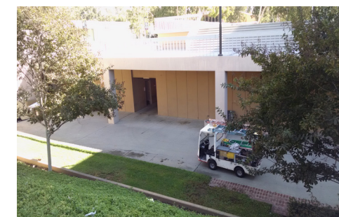
Exhibit 7-9: View into service area from upper level
