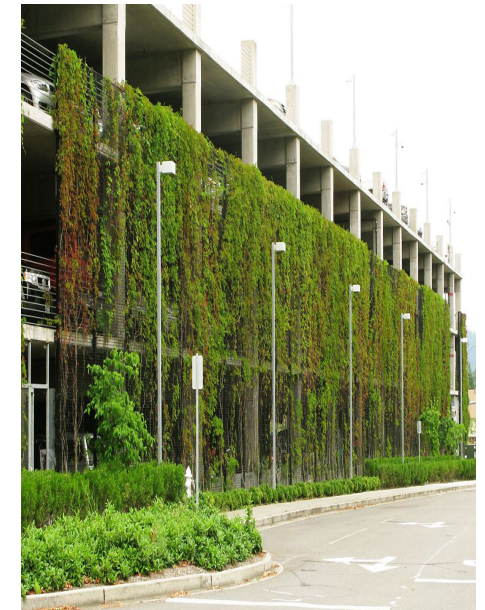
Screen panels planted with vines provide visual relief from an otherwise bare concrete cavernous parking structure.
