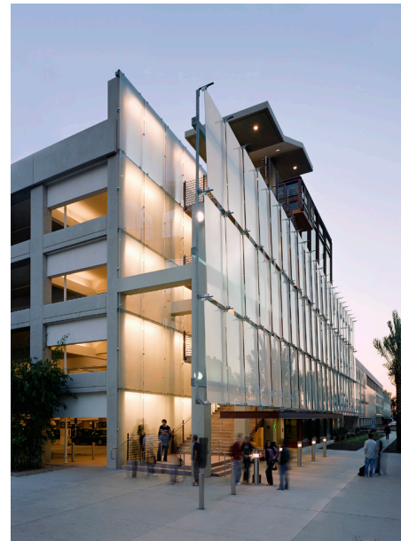
Architectural detailing such as the glass panel treatment shown above can be used to help soften the façade of a parking structure.
