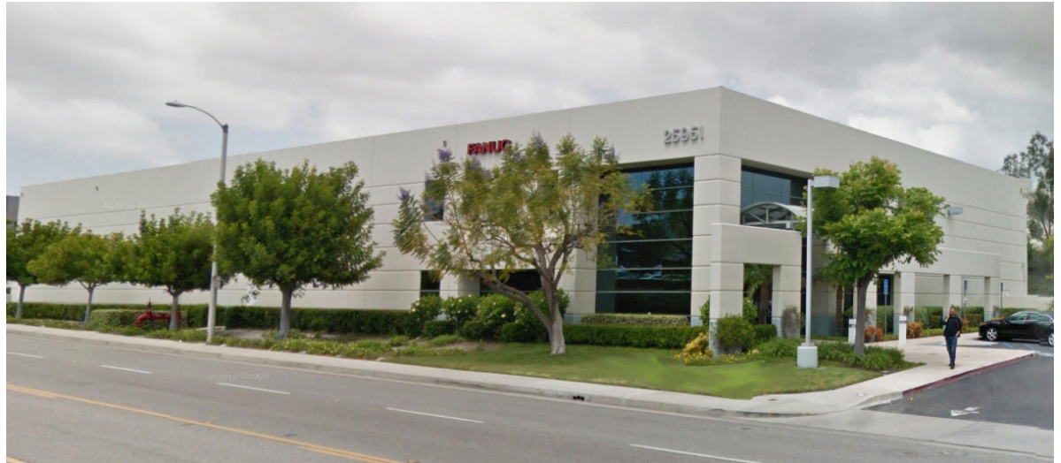
Typical ‘tilt-up’ construction and building type that could be built at University Village along Central Avenue. Note the enhanced features signaling the building entry: Use of glass, concrete screen/arcade and enlarged paved entry with bollard lighting.
