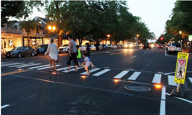
Crosswalks will be an important part of the pedestrian circulation system for the University Village. High visibility continental crosswalks are appropriate for installation at intersections or mid-block with optional lighting alert systems possible for added safety.
